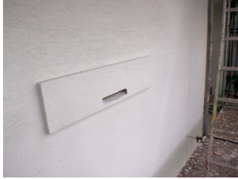
Picture C3-6 (left): Open entrance to roosting site of bats Picture C3-7 (right): Special straight-through-hole batbox through which bats can access their original roosting sites in the crevices between panels
