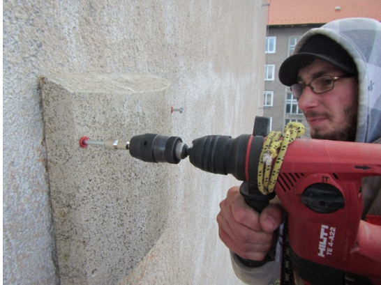
Picture C3-2: Installation of bat boxes suitable for hibernation
