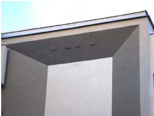
Picture C3-3: Bat boxes implemented in thermal insulation
