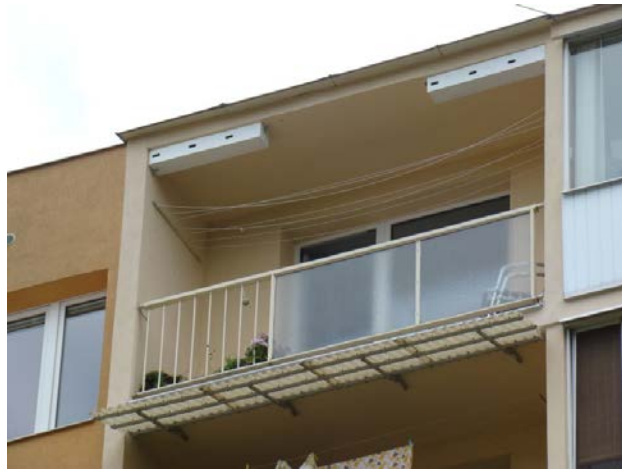
Picture C2-4: Different types of Swift boxes installed on buildings
