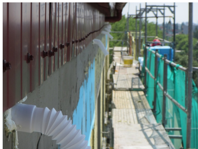
Picture C3-1: Measures for safe displacing of bats from roosting sites in buildings
